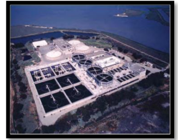
SVCW Regional Treatment Plant
