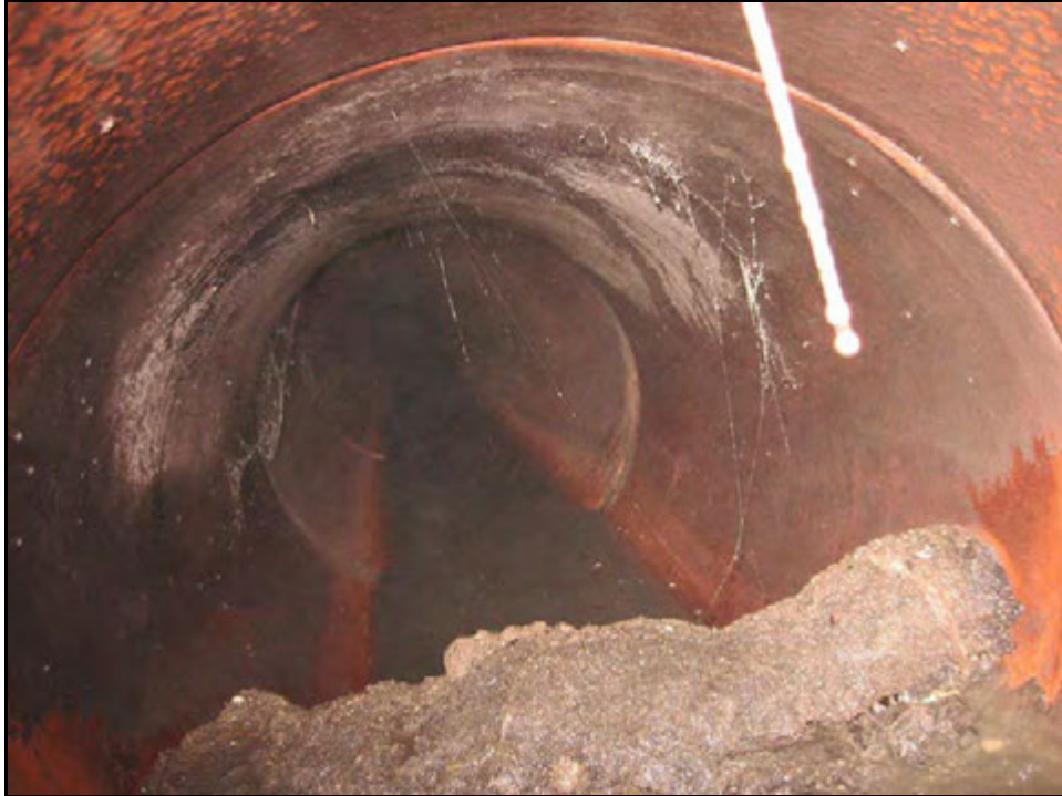
Upstream Overflow Weir
