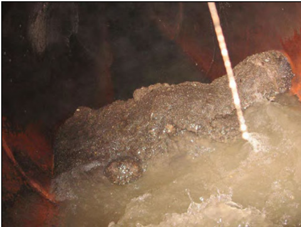
Upstream Overflow Weir
