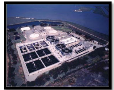
SVCW Regional Treatment Plant
