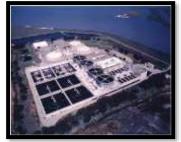
SVCW Regional Treatment Plant
