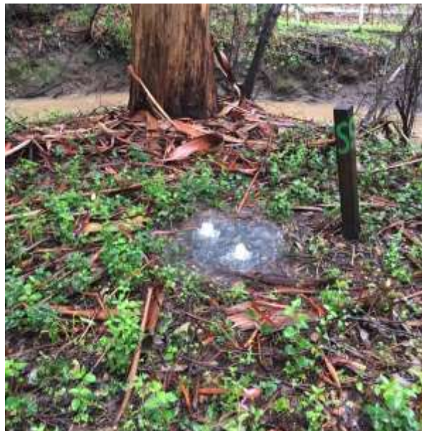
(Example of overflowing manhole)
