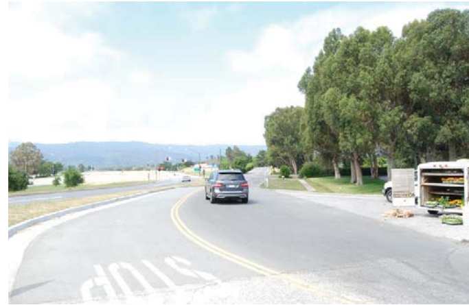
Photo 6. View looking west along the alignment on Sand Hill Road from east of golf course.
