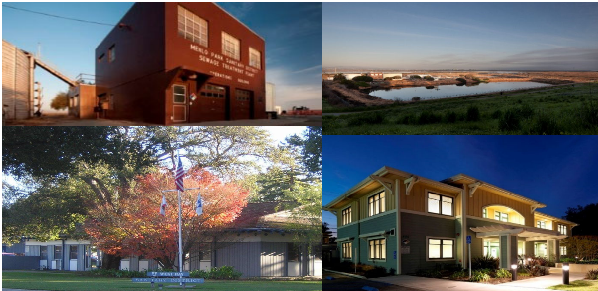
District's old treatment plant, Flow Equalization Pond, 1960 Administration Building, 2009 Administration Building (left to right).
