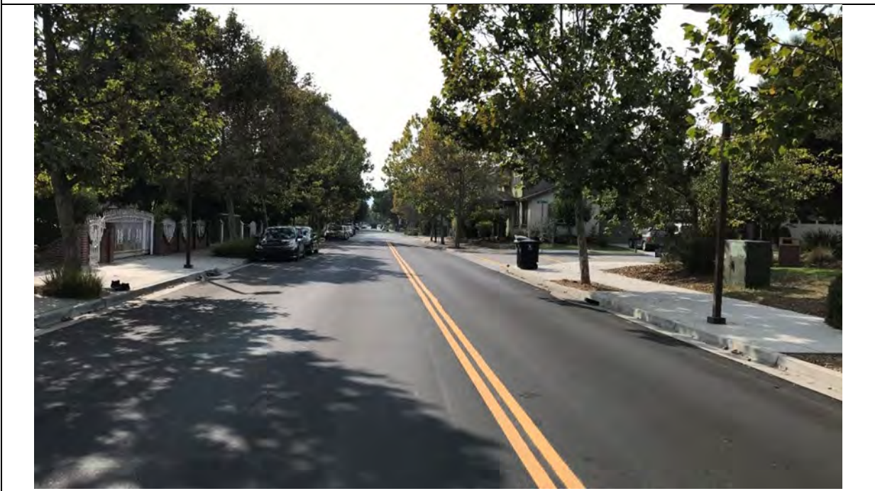
Photo 18. Hamilton Avenue looking west near Hamilton Park.
