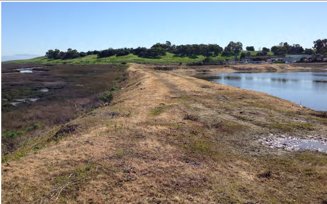
Photo 3. Looking east from the northwest corner of the FERRF property.
