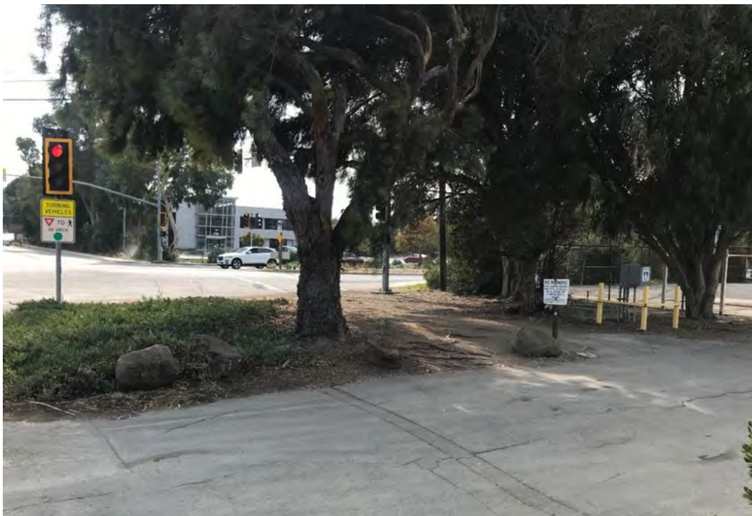
Photo 14. WBSD Influent Pump Station Site.
