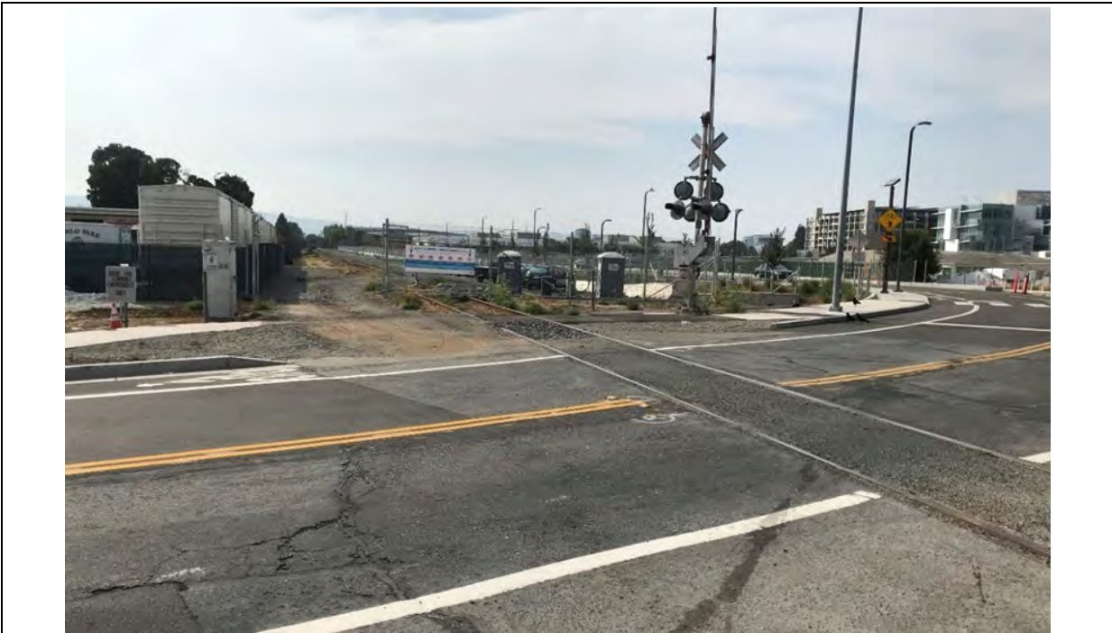
Photo 17. San Mateo County Transit District Rail crossing on Chilco Street looking northwest.
