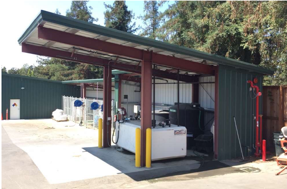
Figure 3.7-1: Existing Metal Canopy
