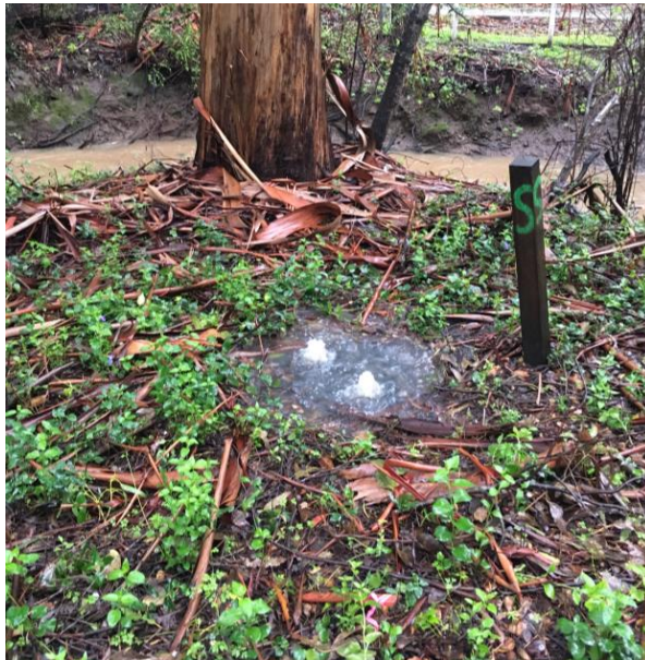
(Example of overflowing manhole)
