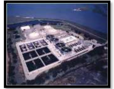
SVCW Regional Treatment Plant
