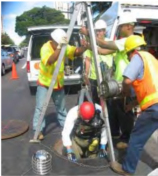
Photo 2-1. Confined Space Entry
