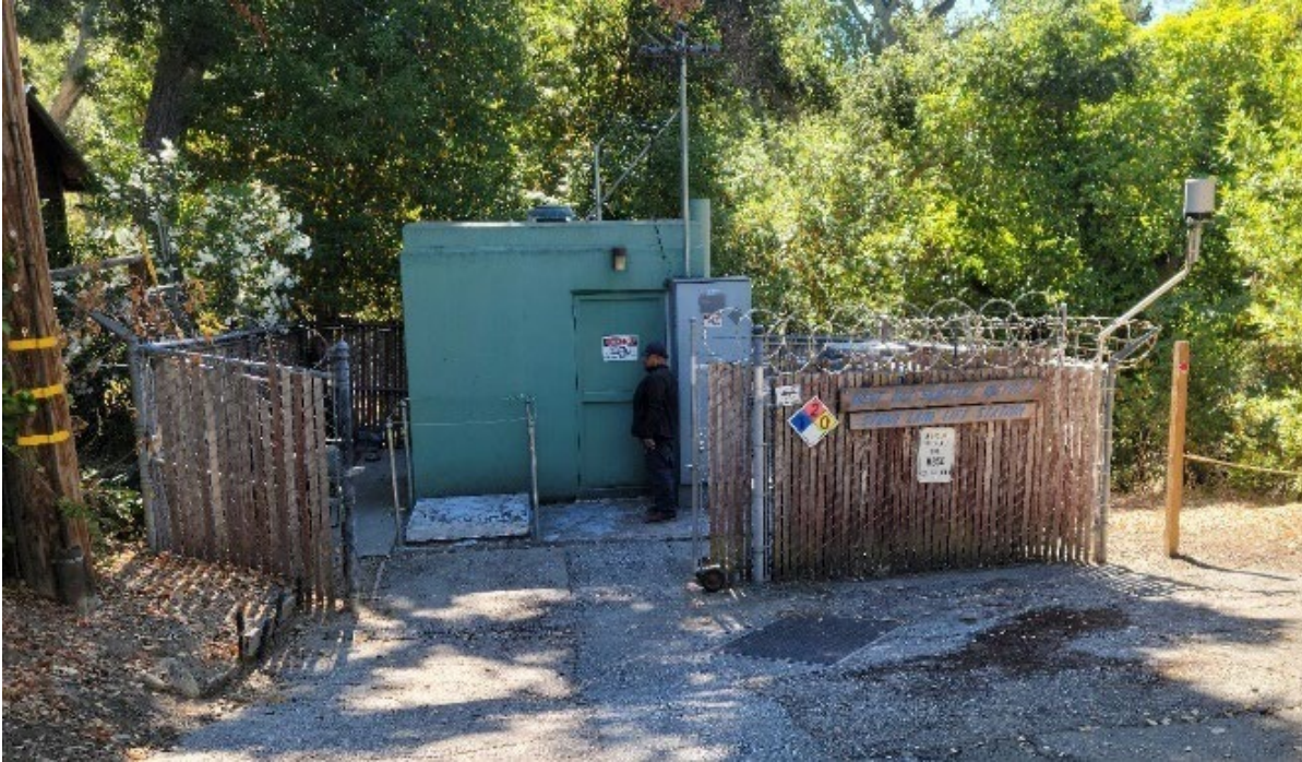
Figure 7.2 – Stowe Lane Pump Station
