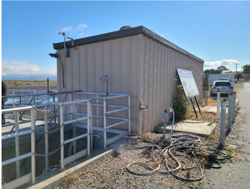
Figure 7.4 FERRF Pump Station
