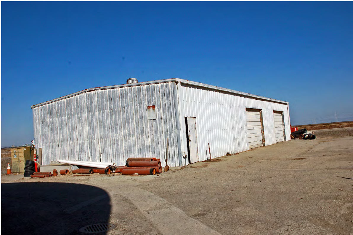
Photo 22. Warehouse. View looking northwest.
