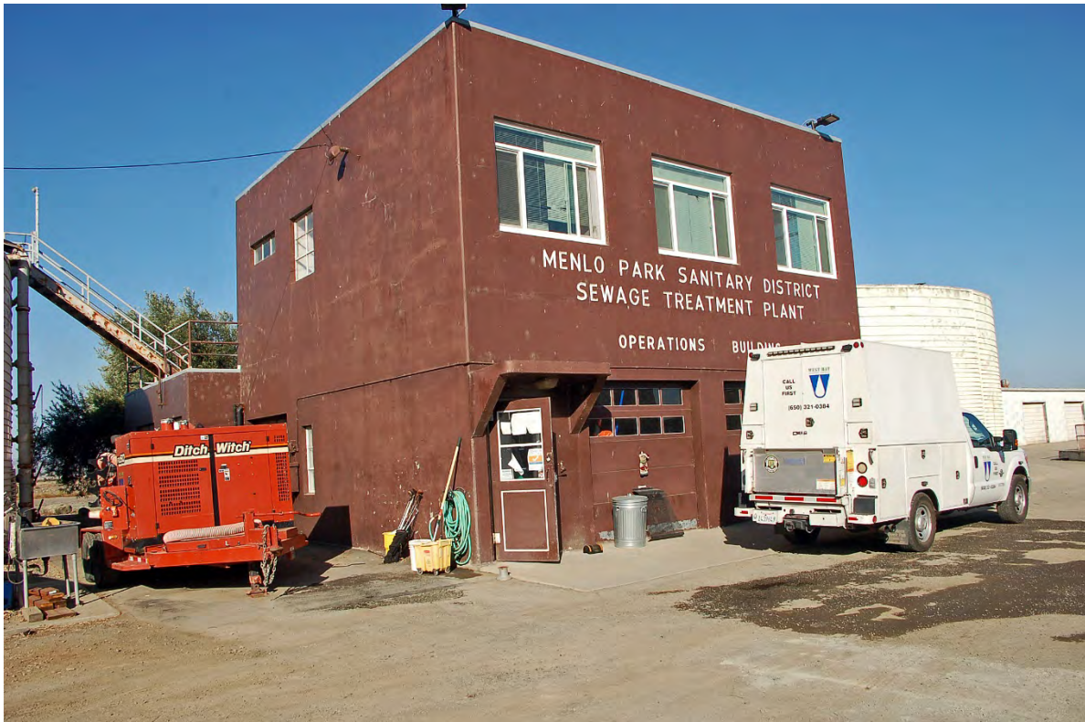
Photo 17. Operations Building. View looking northwest.
