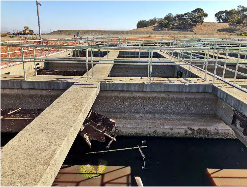
Photos 33. Sedimentation Tanks (1960s). View looking east.
