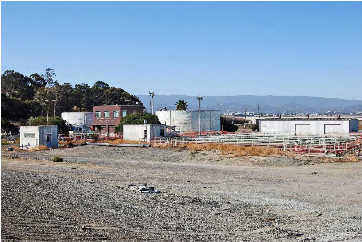
Photo 14. Facilities of the decommissioned Menlo Park sewage treatment plant. View looking west.
