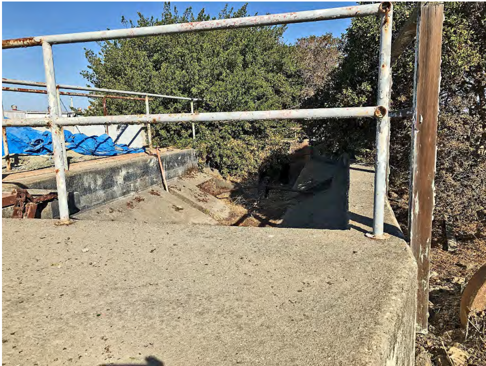
Photo 24. Inlet Works. View looking northwest.
