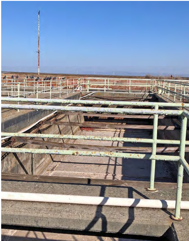
Photo 32. Sedimentation Tanks (1952). View looking north.
