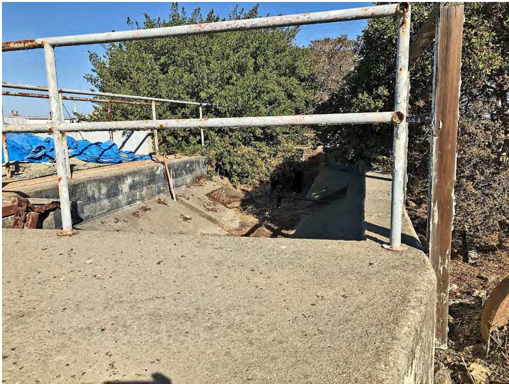
Photo 24. Inlet Works. View looking northwest.
