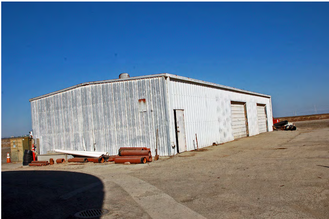
Photo 22. Warehouse. View looking northwest.
