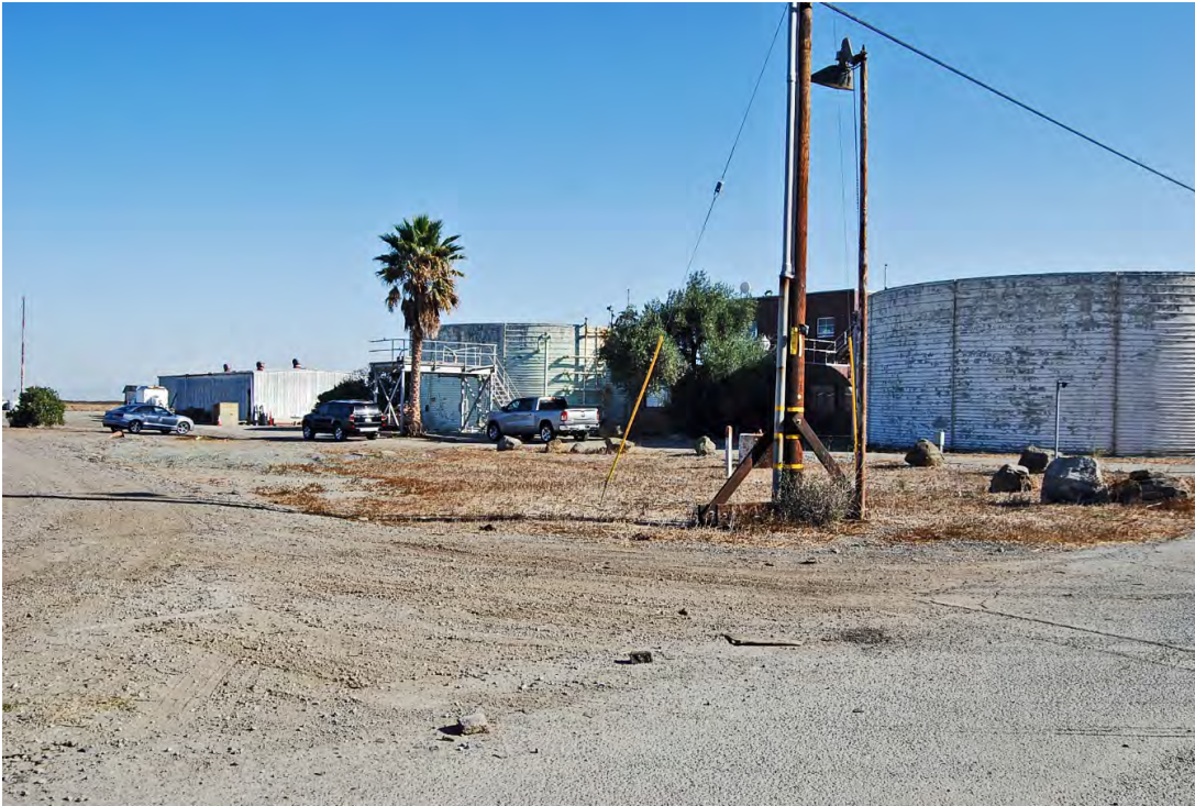
Photo 13. Facilities of the decommissioned Menlo Park sewage treatment plant. View looking northeast.
