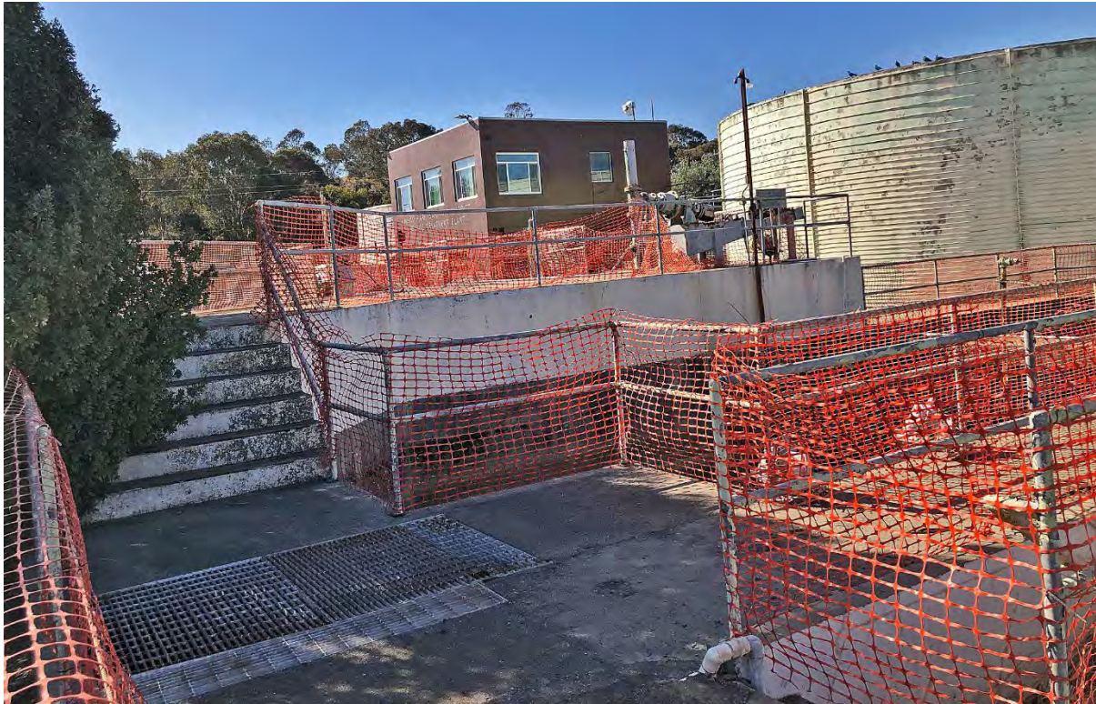
Photo 25. Inlet Works. View looking southwest.
