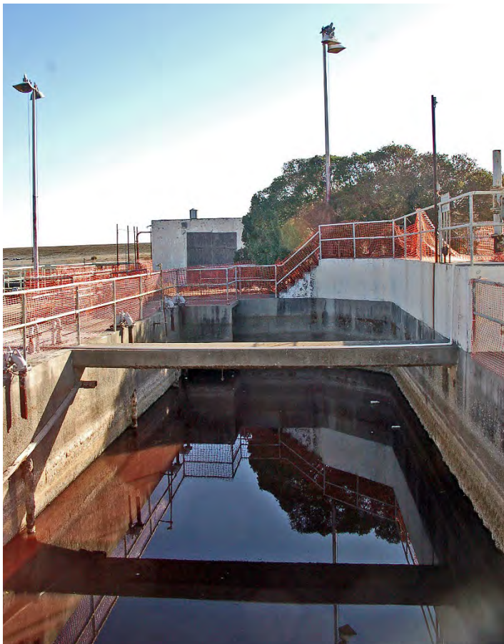
Photo 26. Pre-Treatment Tanks. View looking east.
