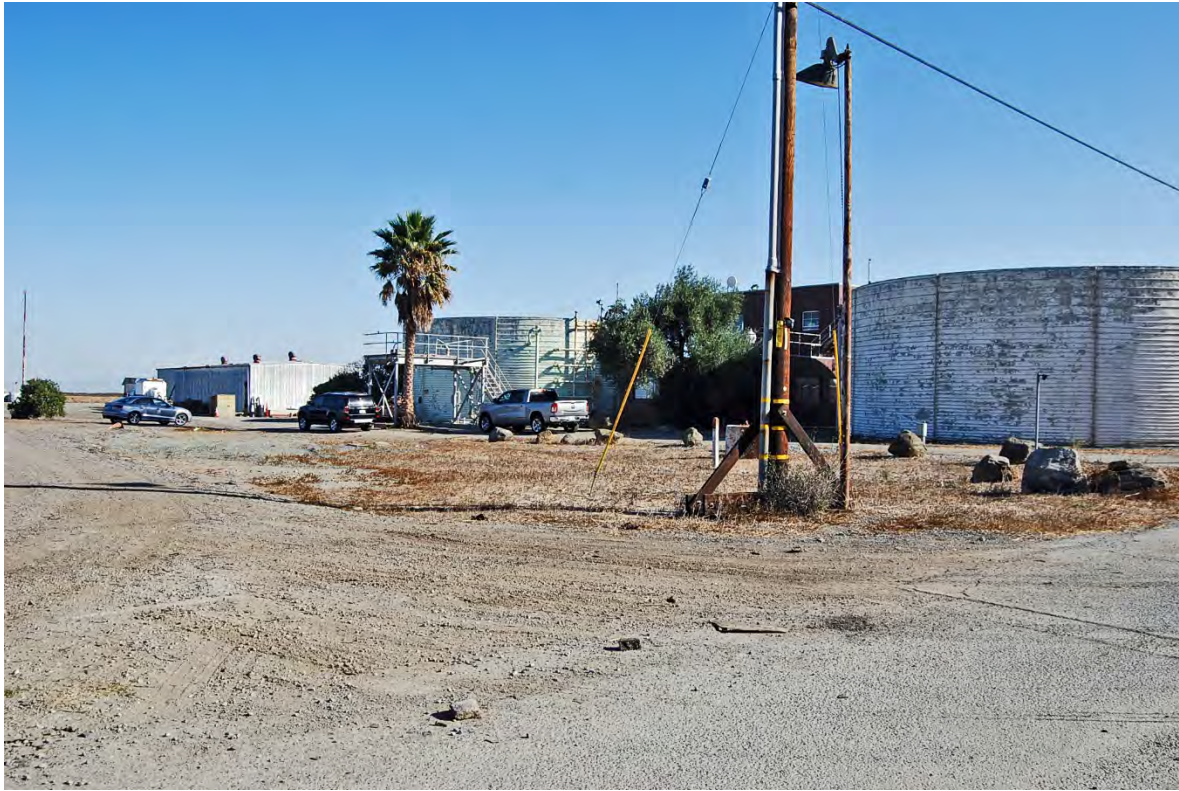
Photo 13. Facilities of the decommissioned Menlo Park sewage treatment plant. View looking northeast.
