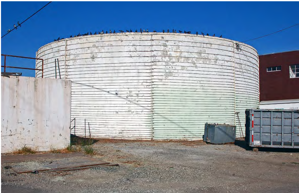
Photo 16. Digester No. 1. View looking northwest.
