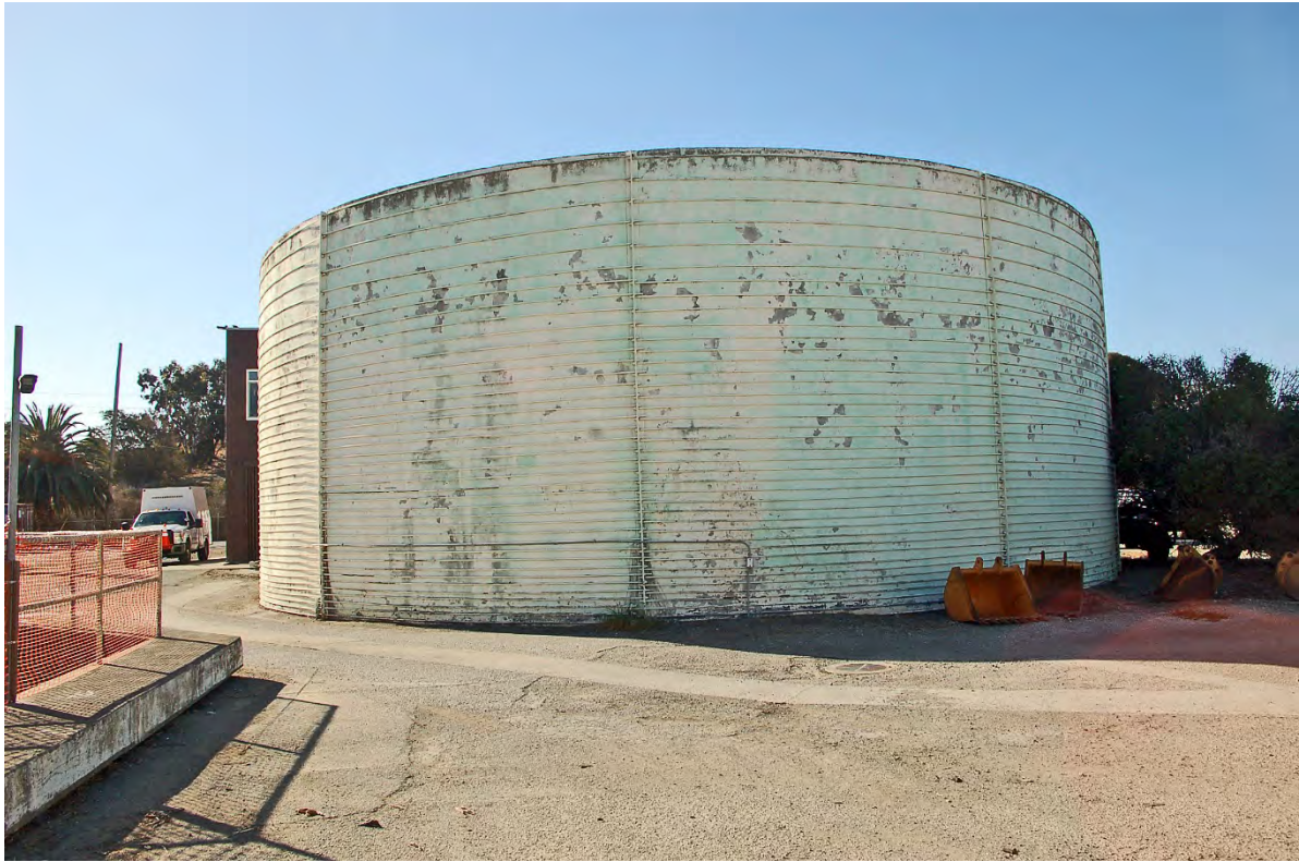
Photo 21. Digester No. 2. View looking southwest.
