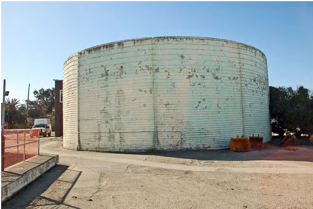
Photo 21. Digester No. 2. View looking southwest.
