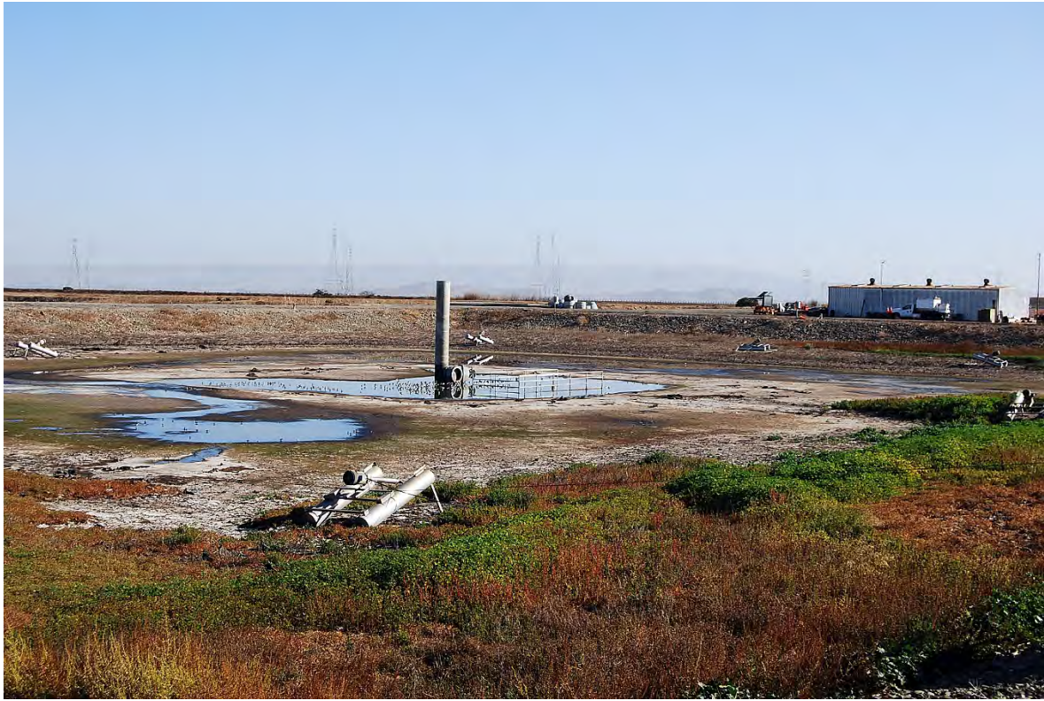
Photo 4. Pond 1. View looking northeast.
