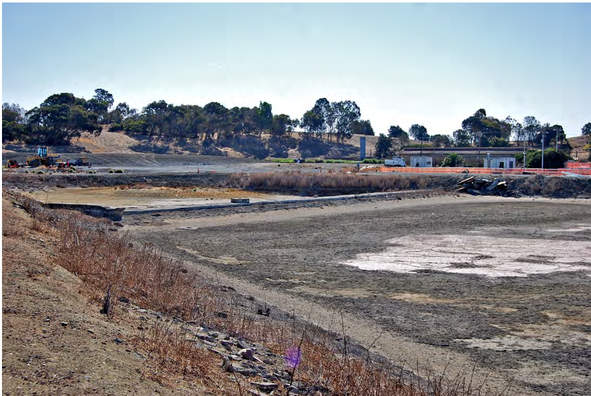
Photo 10. Pond 3. View looking southeast.
