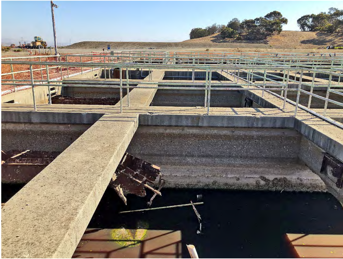
Photos 33. Sedimentation Tanks (1960s). View looking east.
