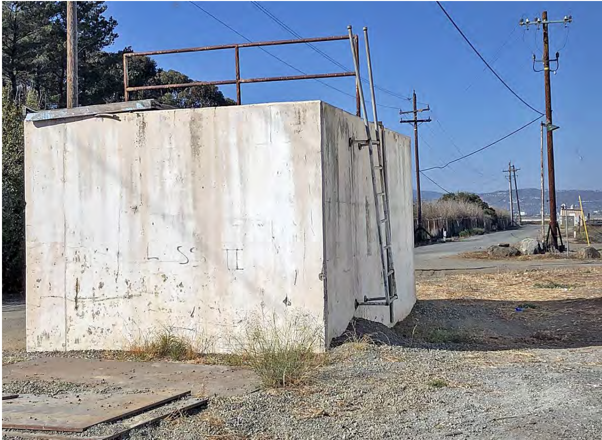
Photo 15 Diversion Box. View looking west.
