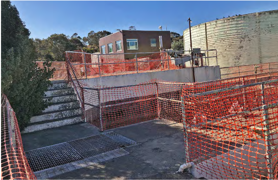
Photo 25. Inlet Works. View looking southwest.
