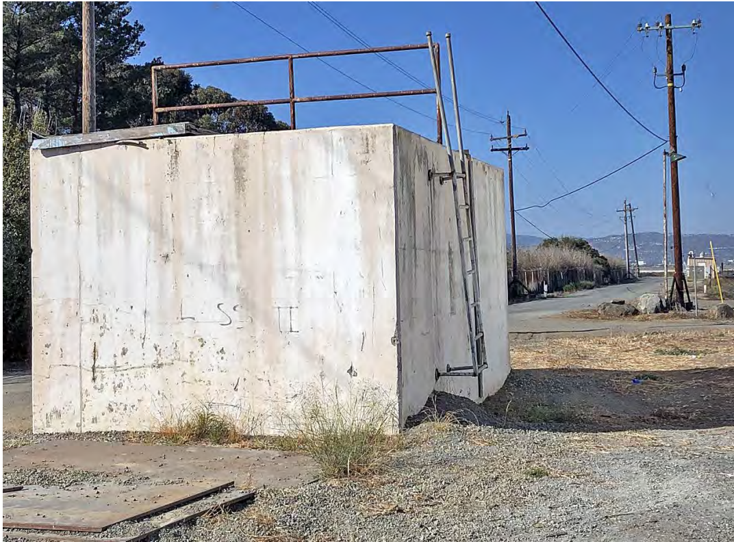
Photo 15 Diversion Box. View looking west.
