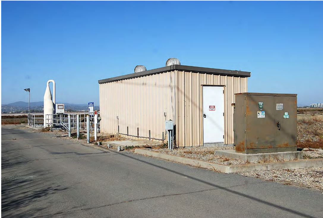
Photo 3. Return pump station. View looking northwest.
