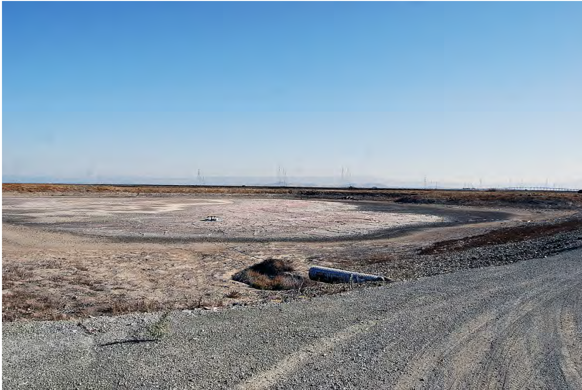
Photo 5. Pond 2 showing pipe connection to Pond 1. View looking northeast.
