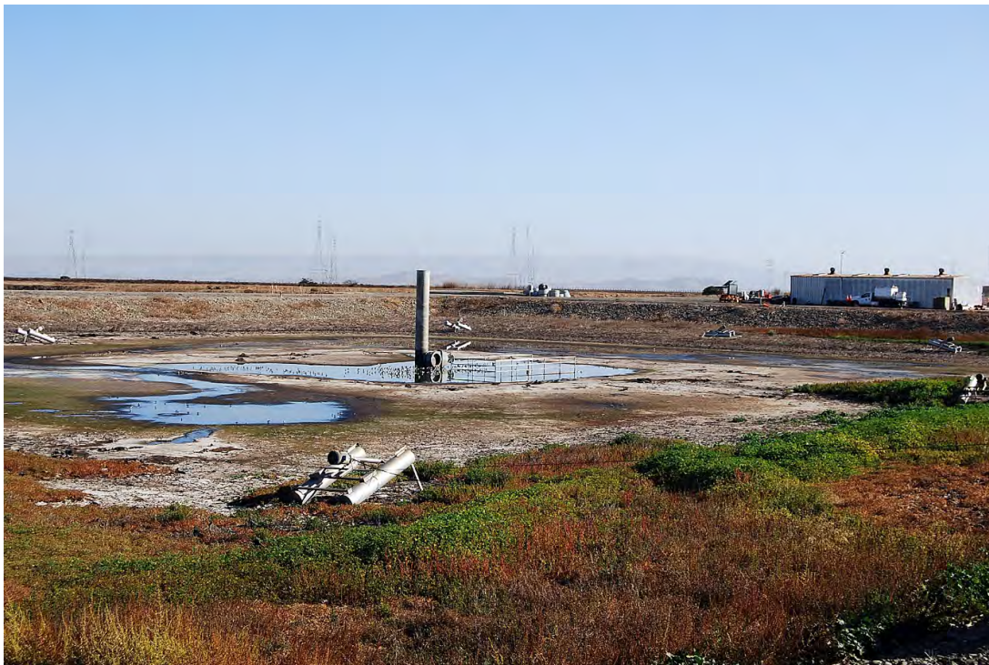
Photo 4. Pond 1. View looking northeast.
