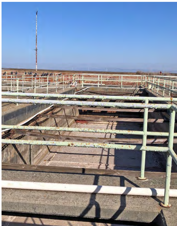
Photo 32. Sedimentation Tanks (1952). View looking north.
