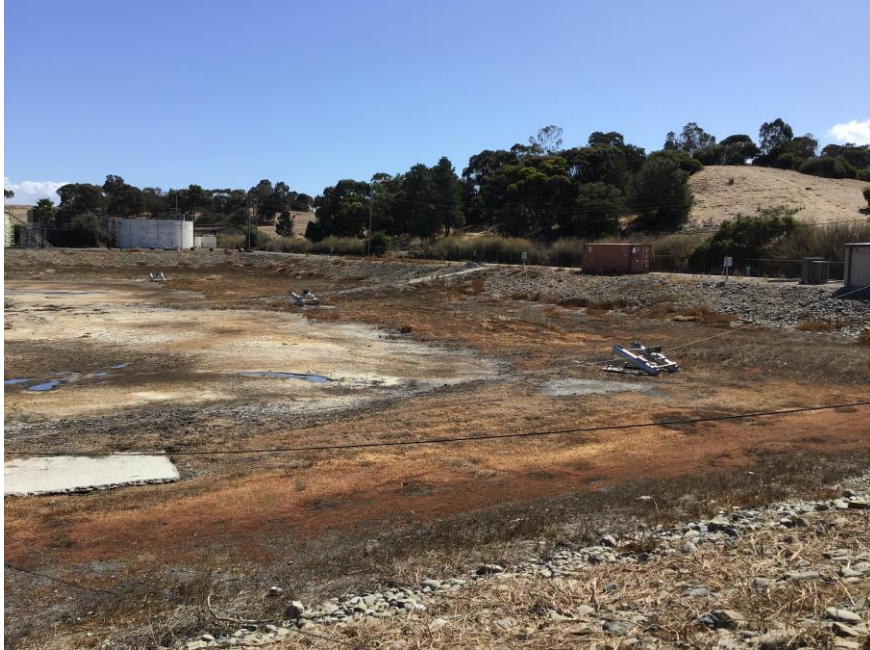
Photo 3. Detention pond within the study area.
