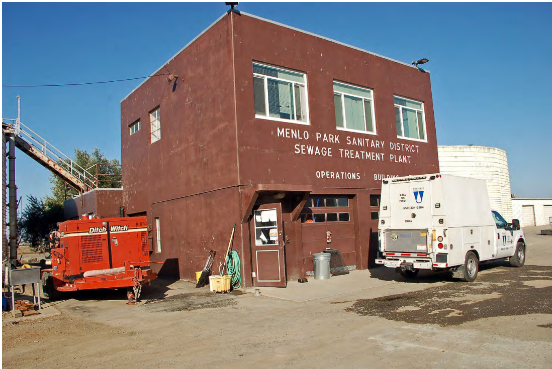
Photo 17. Operations Building. View looking northwest.
