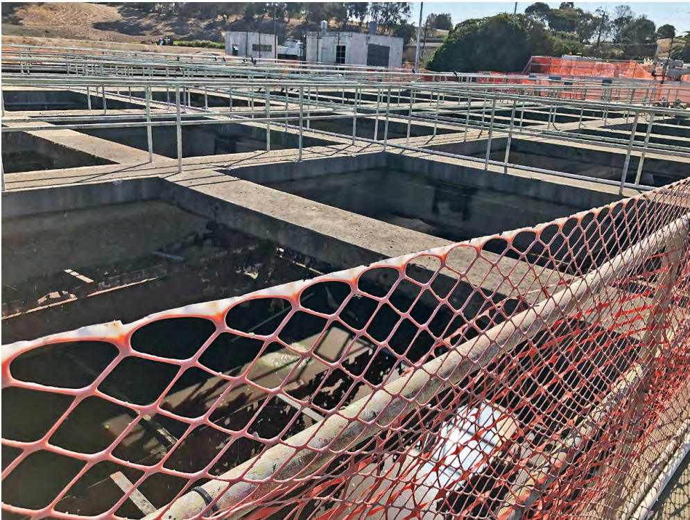
Photos 34. Sedimentation Tanks (1960s). View looking southwest.
