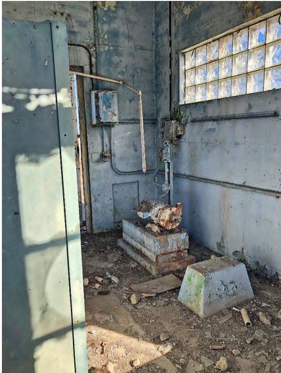
Photo 31. Chlorination Building. Interior view.
