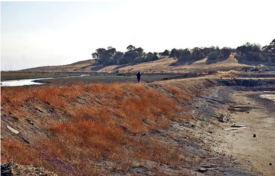
Photo 8. Levee and dirt road along the north side of the FERRF property. Levee provides separates the property from Westpoint Slough (left) and forms the north side of Pond 2 (right foreground) and Pond 3 (right background). View looking east.
