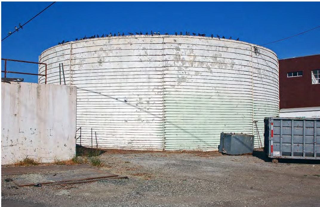
Photo 16. Digester No. 1. View looking northwest.
