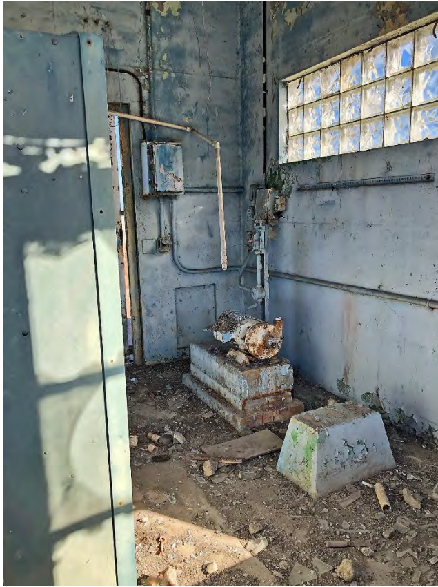
Photo 31. Chlorination Building. Interior view.
