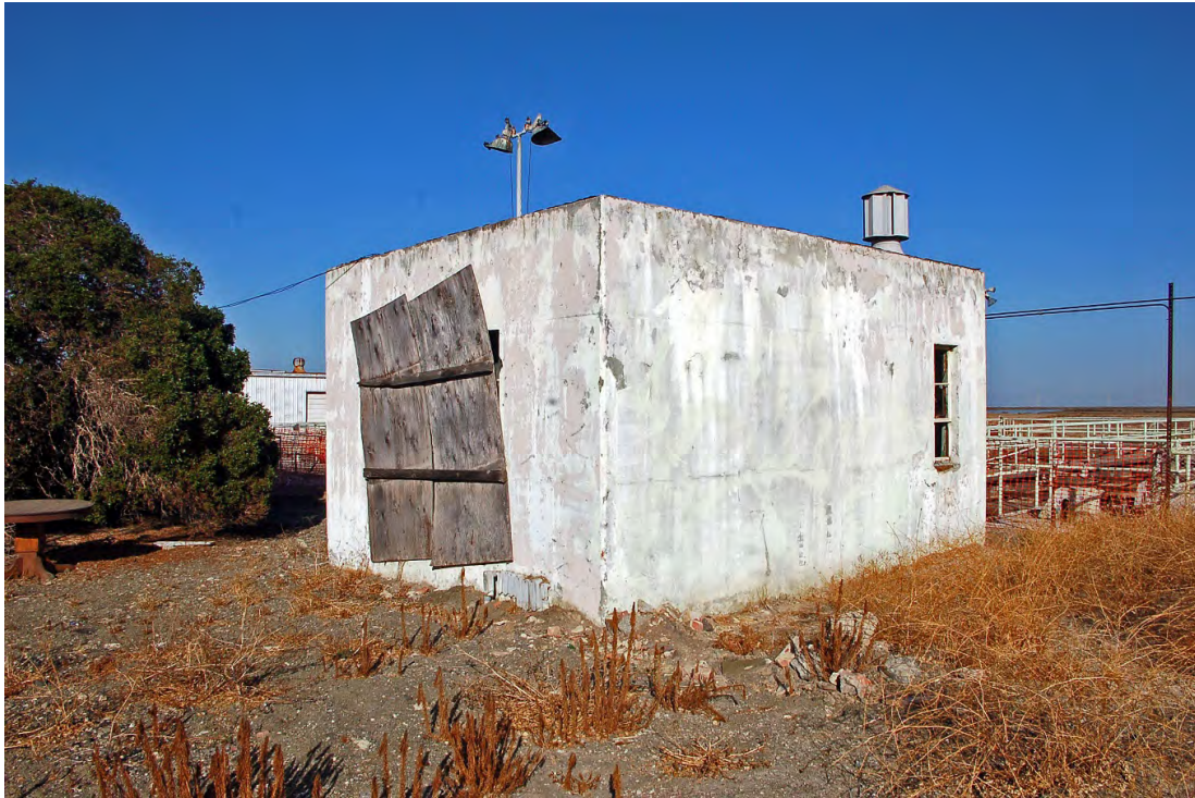
Photo 27. Pump House: View looking northwest.
