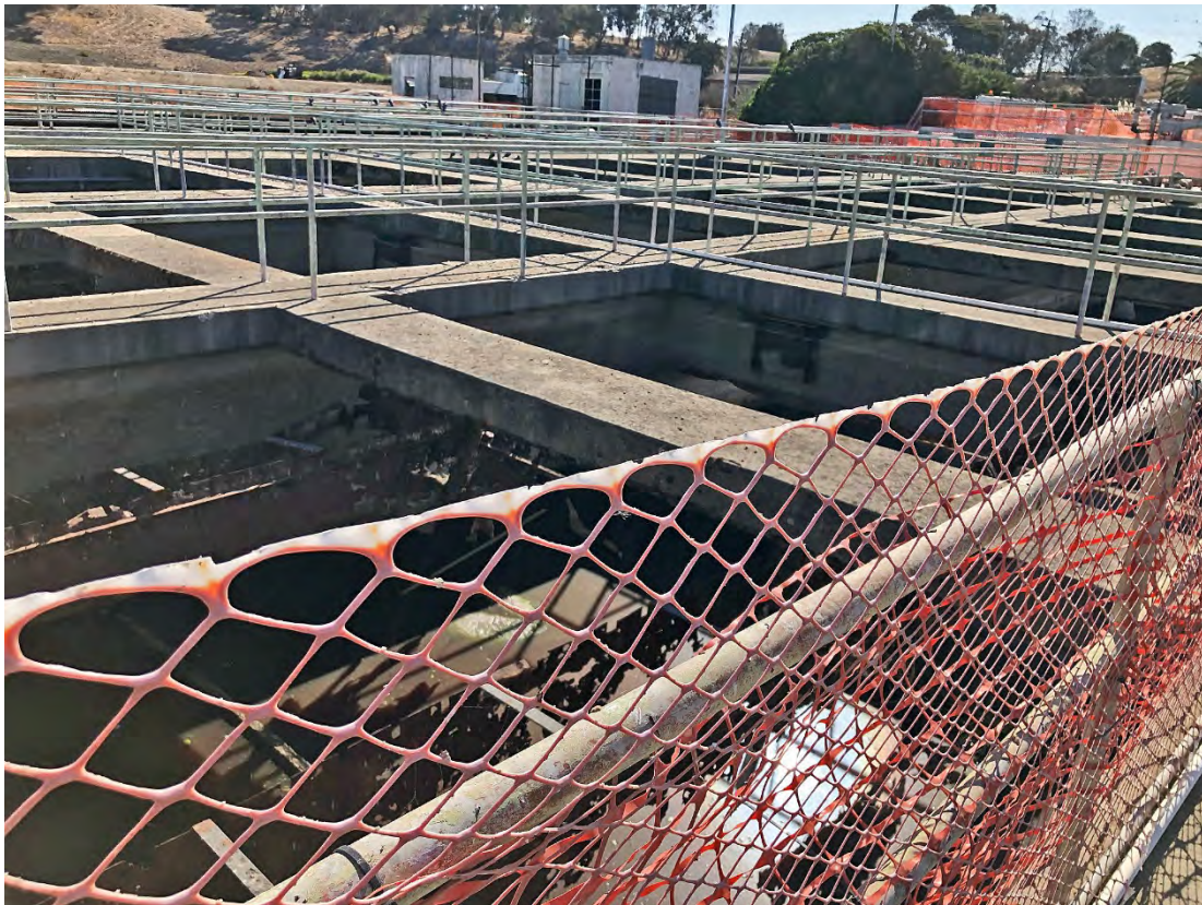
Photos 34. Sedimentation Tanks (1960s). View looking southwest.
