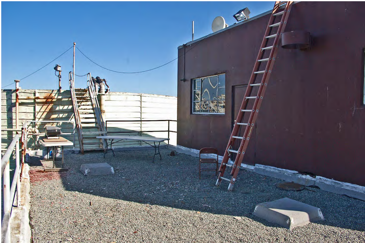
Photo 18. Operations Building. Rear stair to Digester No. 2. View looking north.
