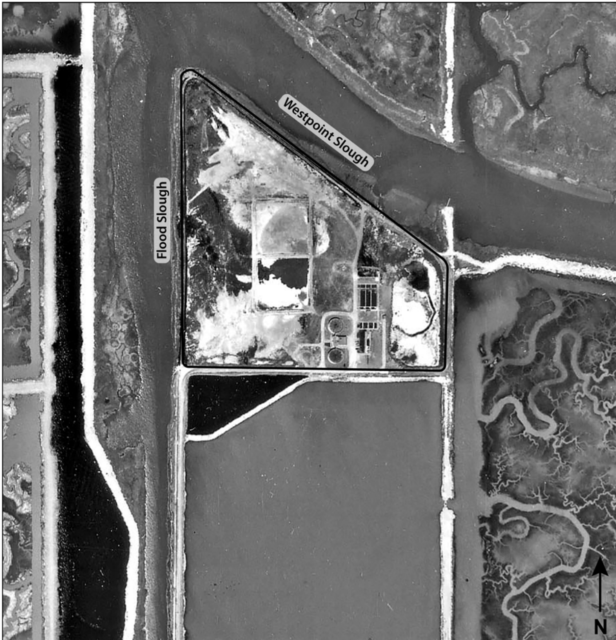
Figure 3. Menlo Park Sanitary District Sewage Treatment Plant in 1955 (Source of Base Map: Pacific Aerial Surveys 1955)
