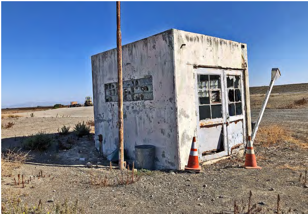
Photo 30. Chlorination Building. View looking northeast.
