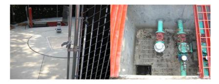
Required equipment for by-passing this station, <u>6-inch trash pump</u>, **6**" suction hose & **4**" discharge hose, 2-6"X4" female to male camlocks. (4" By-Pass)
