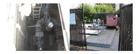
Required equipment for by-passing this station, 6-inch trash pump, 6"suction & discharge hose (6" By-Pass).
