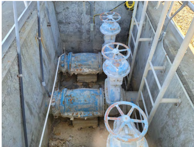
Figure 7.5 FERRF Pump Discharge Valves
